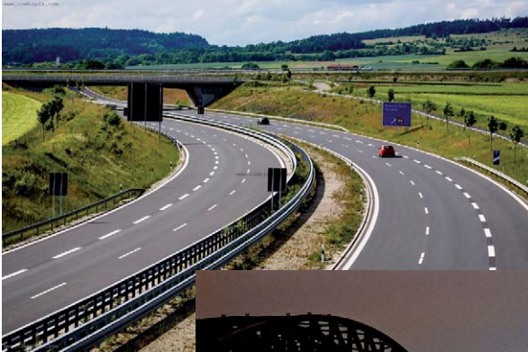
highways in Germany
